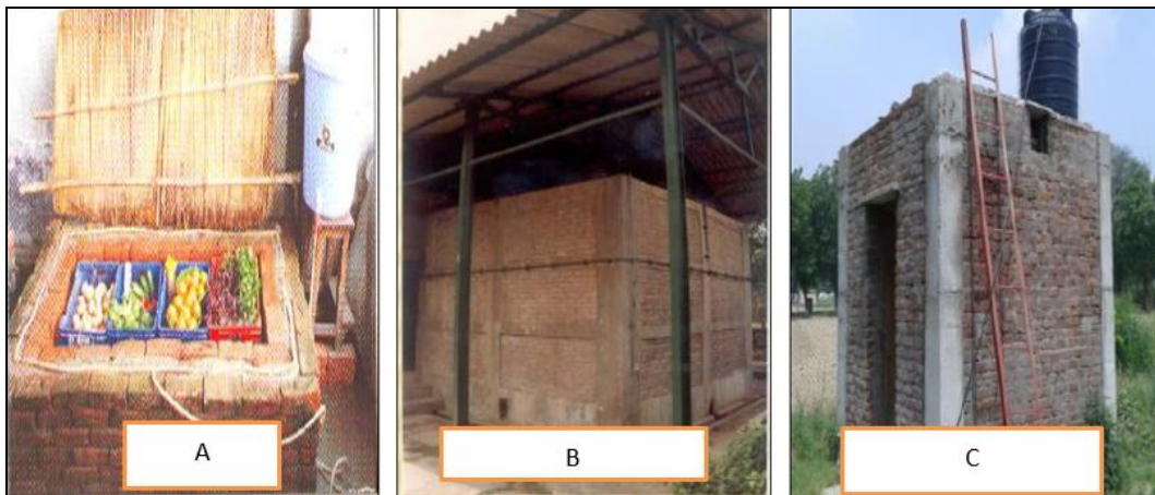
Fig 3: Evaporative cool chamber (ECC) (A) and improved ECC (B and C);Source kale et al. , 2016
